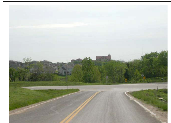
E 1500 Rd & K-10 – looking east toward Lawrence.
