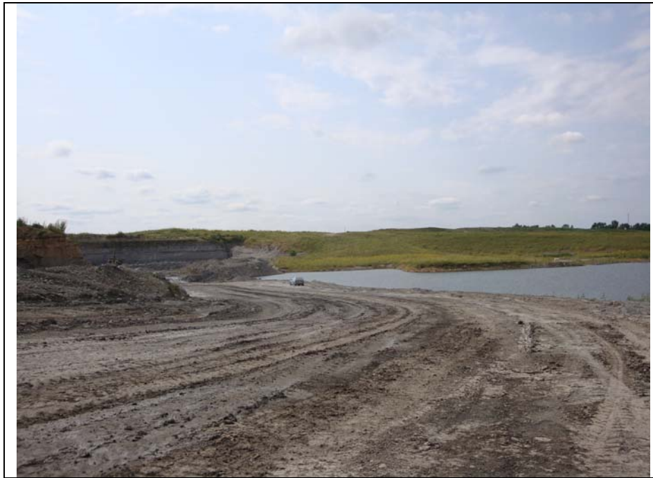
Figure 11. Work being done to reshape the water feature in Phase 1A.
