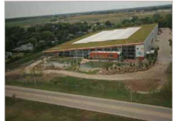
Aquascapes Green Roof, St. Charles, IL
