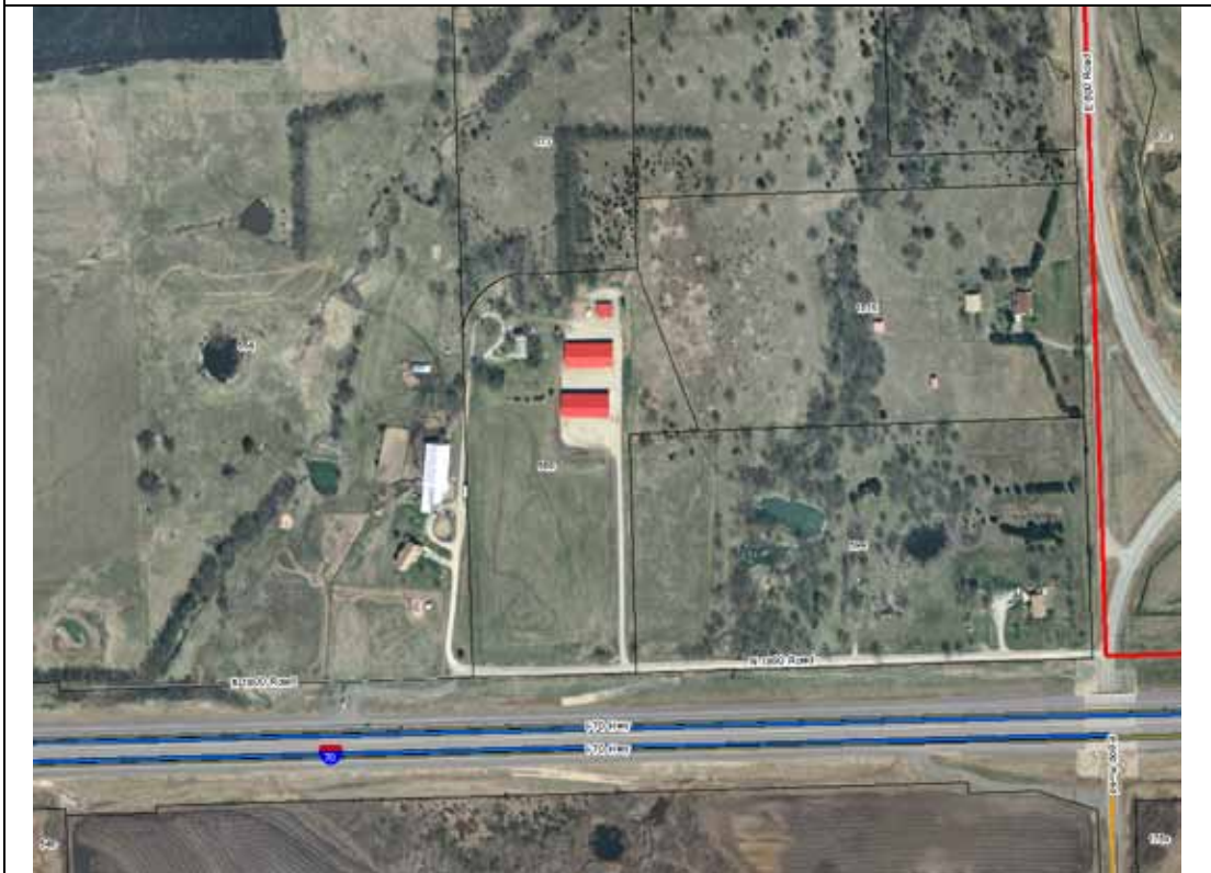
Figure 1b. This detail shows the buildings in relation to the adjacent roadways. N 1800 Road ends at property to west.
