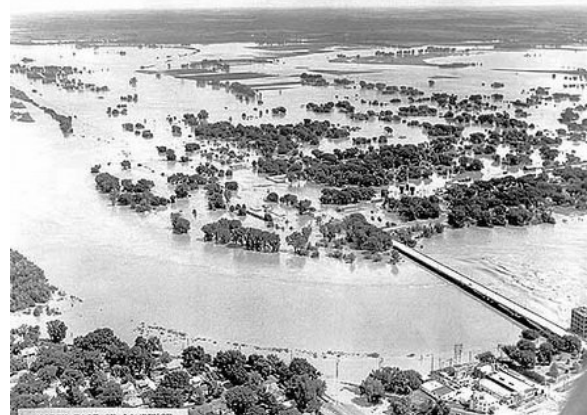
Figure 6 - View of the 1903 Flood, UP Depot spire visible in the distance, Bowersock Power Plant at the far right, from F.M. Knight Booklet "Views of the Great Kansas River Flood – Lawrence". And aerial view of the 1951 Flood, Lawrence Journal World, file photo.
