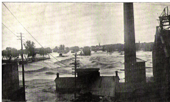
VIEW BELOW MILL DAM LOOKING OVER ELECTRIC LIGHT PLANT WITH PART OF NORTH LAWRENCE IN DISTANCE.
