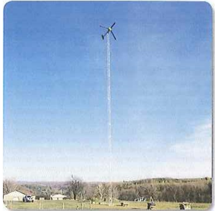
A residential 10 kW turbine on 140-foot freestanding lattice tower.
