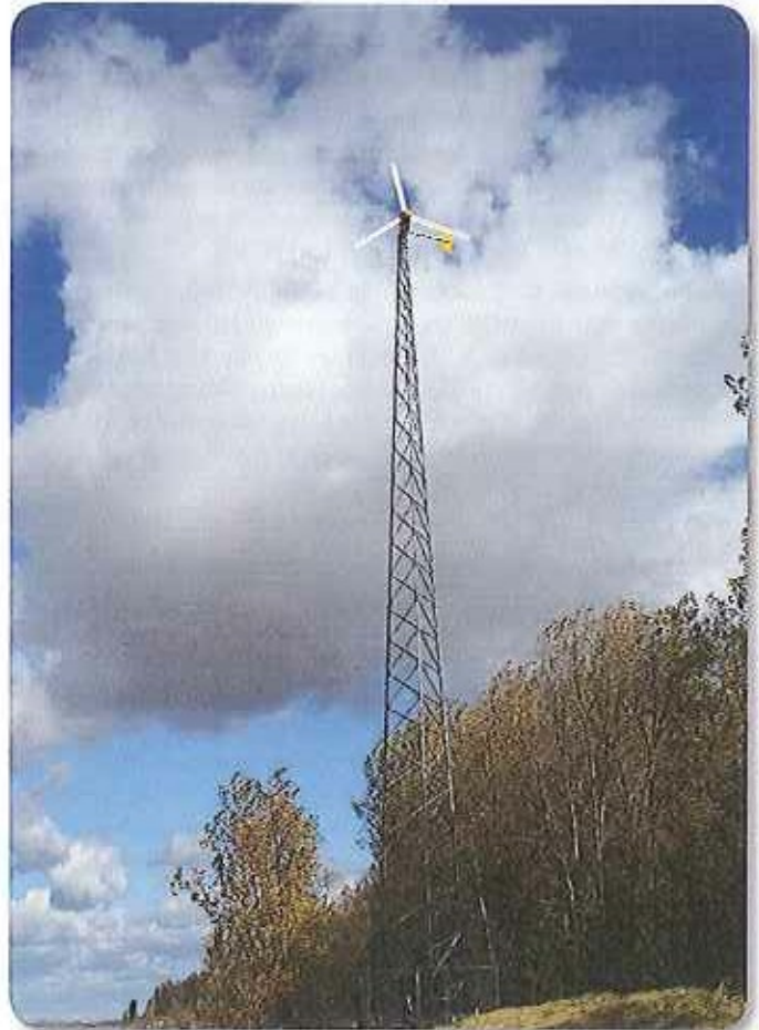
A 10 kW, 140 ft. freestanding lattice tower at a state park.
