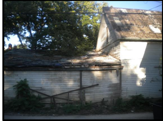
Rear of Garage
