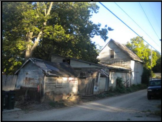
Rear of Shed/Garage/Barn
