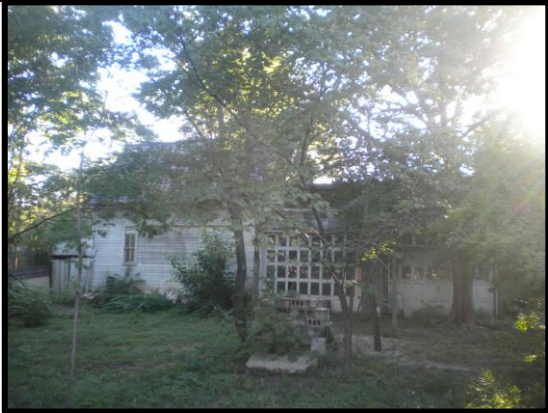
Front of Garage/Barn
