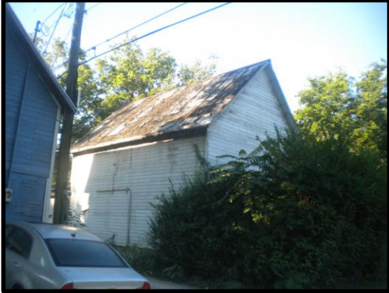
Rear of Barn
