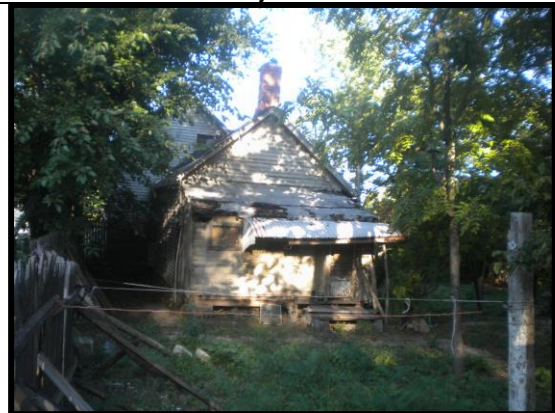
Rear of Subject
