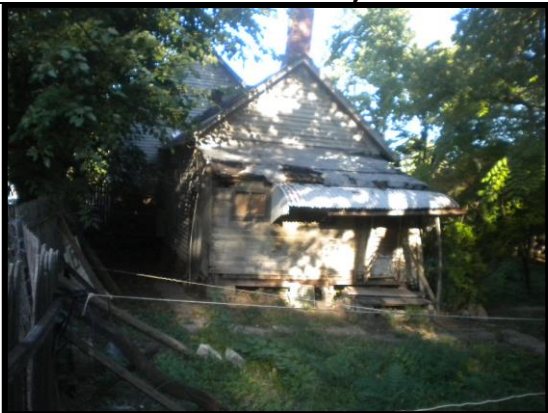
Rear of Subject
